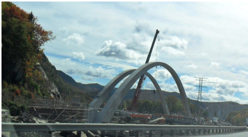
Arch bridge, Route 175 in Stoneham ↑↑
