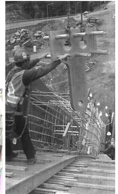
Arch bridge, Route 175 in Stoneham ↑↑
